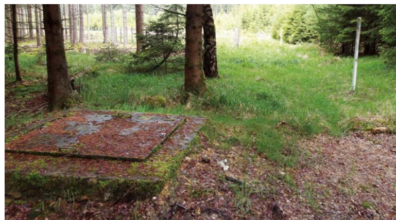
Fig. 7. No water flows at the surface from the captured Pekelský stream spring near Aš, which is enclosed in a chamber (photo: P. Eckhardt)
