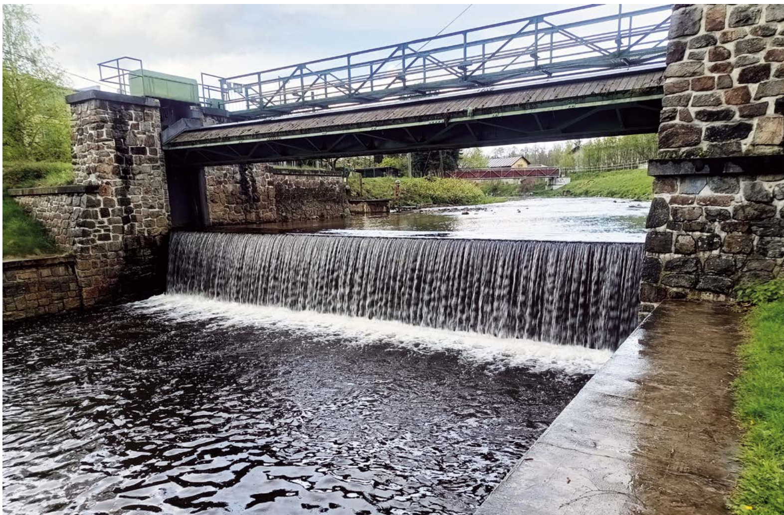
Fig. 3. Current condition of the fixed weir with a movable gate in Rybáře at river km 1.1 (photo: E. Bouše)
