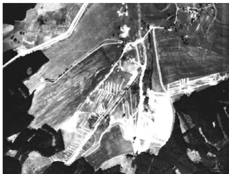
Fig. 8. Historical aerial photograph showing the construction of drainage systems around the village of Pastviny in the Aš area
