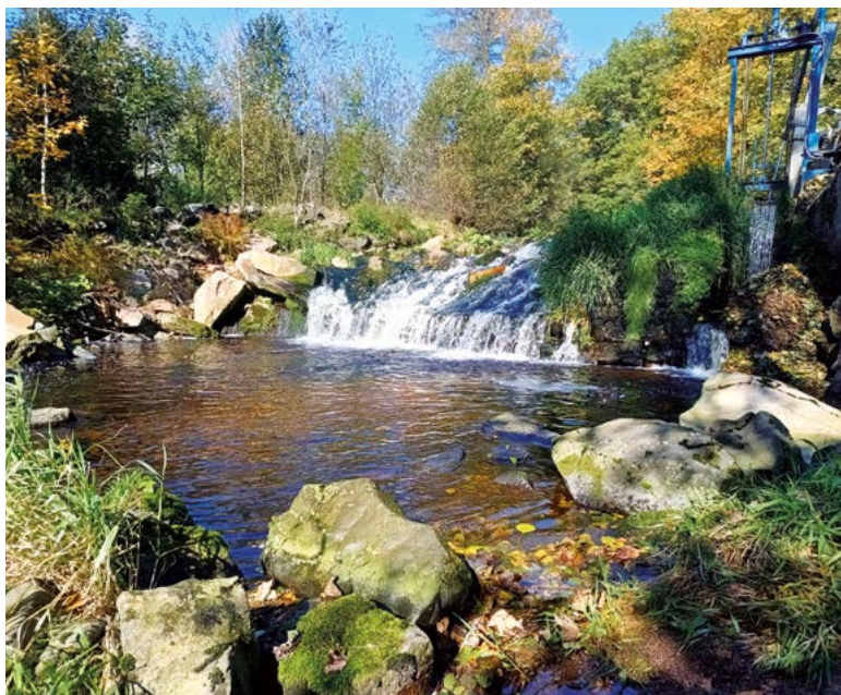
Fig. 4. Weir in Stará Role at river km 4.6, constructed of boulders embedded in concrete (photo: E. Bouše)
