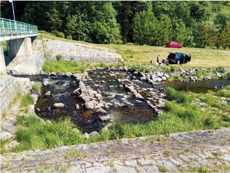
Fig. 6. Restored weir in Nová Role at river km 9.2 (photo: E. Bouše)
