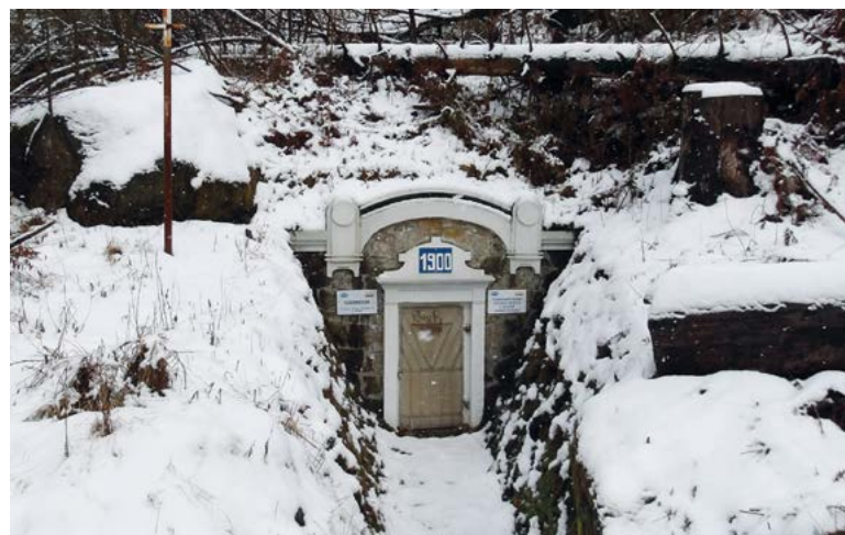
Fig. 4. Historical capture structure at Nad Klepáčem spring near Hřensko; condition in February 2026 (photo: P. Eckhardt)
