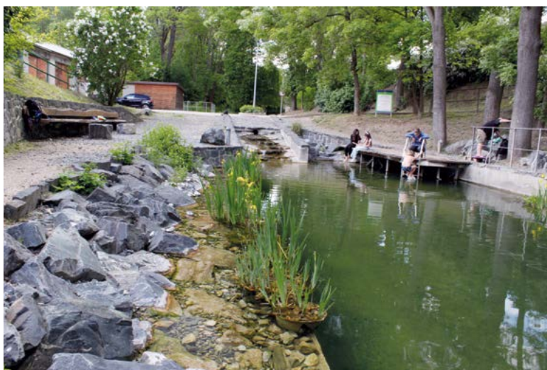
Fig. 5. Revitalisation of the fire pond on the Lysolaje stream and the upper section of its channel below one of Prague's most productive springs, the so-called Miraculous Spring (Zázračná studánka). The recreational biotope is now fed by this spring, making it one of the coldest water bodies in Prague
