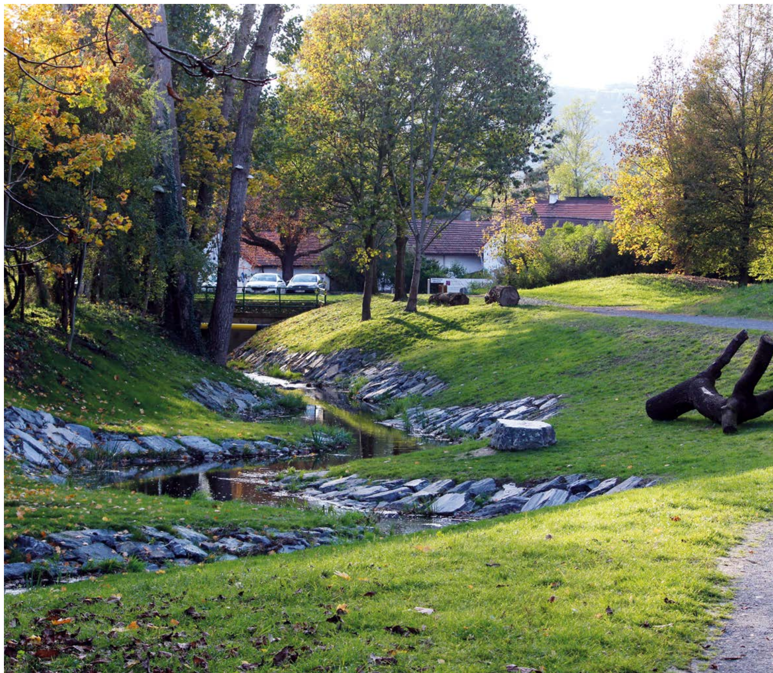
Fig. 7. Revitalisation of the lower reach of the Kunratice stream in Braník, in Za mlýnem Park, commissioned by the Prague City Hall (construction supervision) in cooperation with the Prague 4 Municipal District. This extensive restoration project also incorporates the use of decorative boulders and large woody debris
