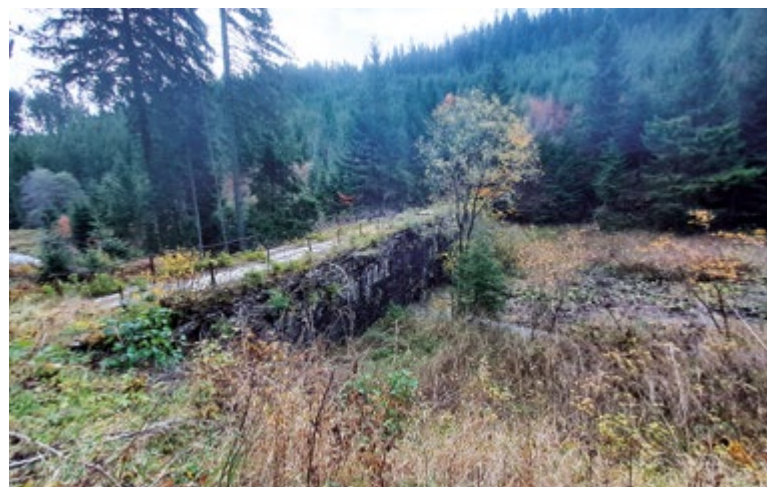
Fig. 13. Upstream slope of Magurka splash dam, November 2025
