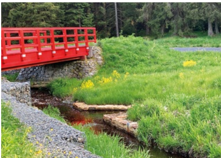
Fig. 6. Blatenský Water Ditch with a newly repaired footbridge (June 2025)
