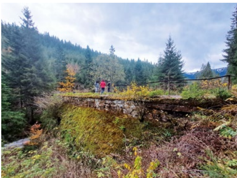
Fig. 12. Downstream slope of Magurka splash dam, November 2025
