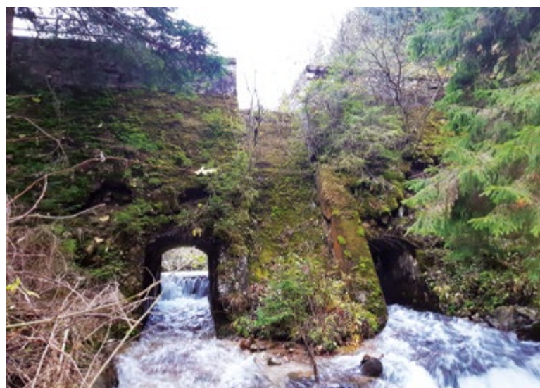
Fig. 14. Relics of outlet galleries of Magurka splash dam, November 2025
