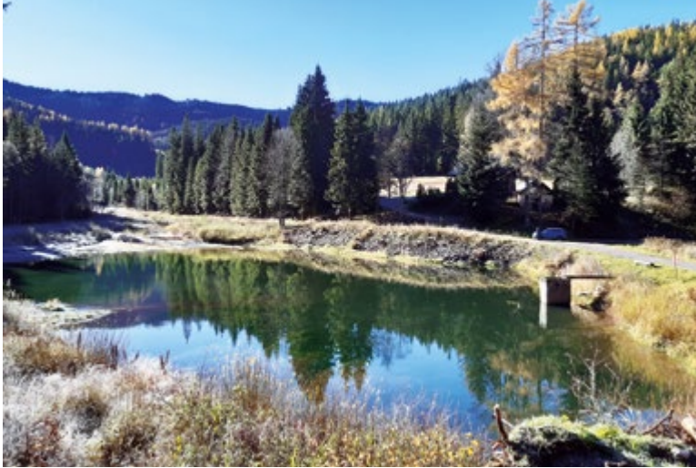
Fig. 7. Malužiná splash dam (right) and reservoir (view from the east), November 2025
