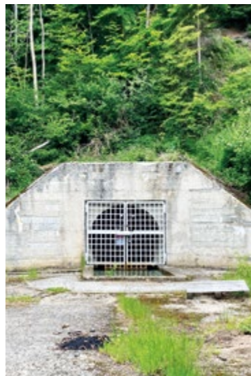
Fig. 24. New drainage adit
