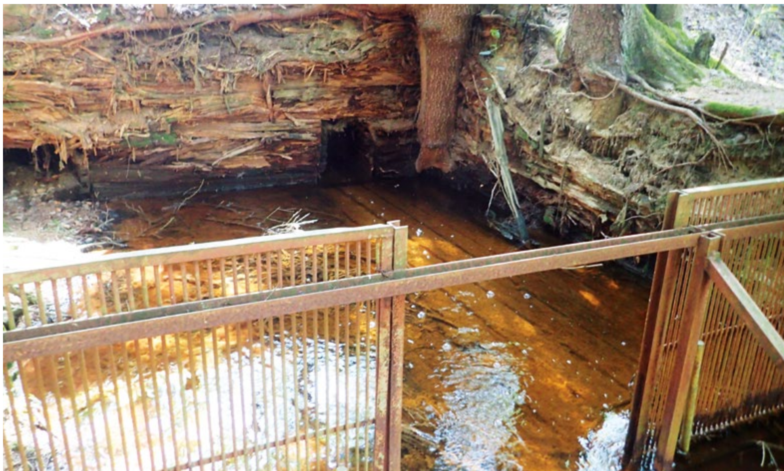
Fig. 3. Remains of a wooden outlet pipe at Huťský pond (photo: M. Bureš, July 2024)
