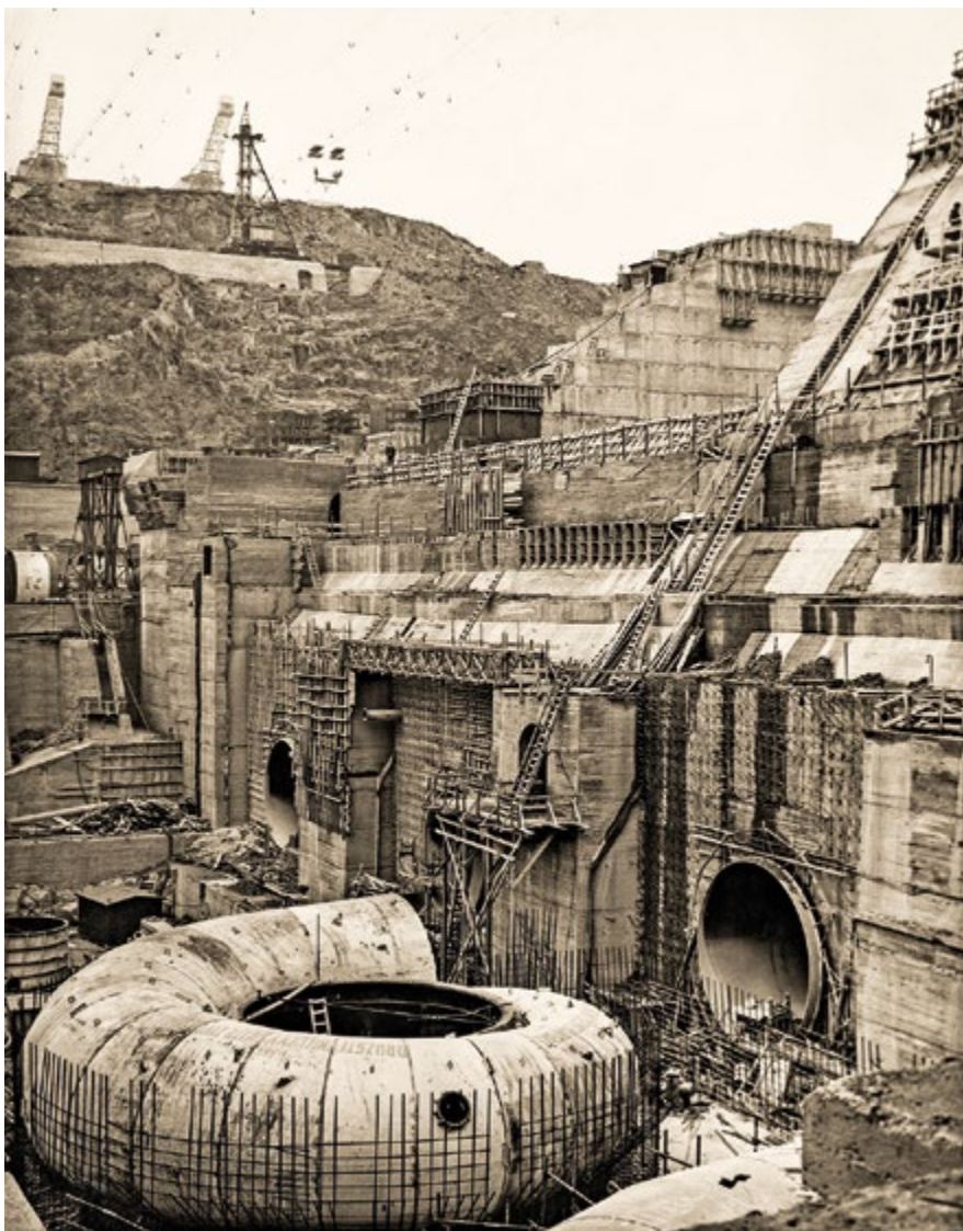
Orlík hydraulic structure is the highest and most massive structure in the cascade of Vltava reservoirs. Its 450 m long concrete dam reaches a height of 91 m at the crest. The Water Research Institute determined the design of the spillway and stilling basin through model testing. The properties of the intake gates for the power station and the thermal regime of Orlík Reservoir were also examined using physical models. From the construction of Orlík Dam (4 November 1959).
