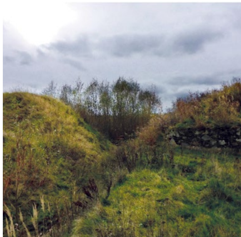
Fig. 6. The gap in Mlékovický Pond dam and the state of vegetation in the flooded area four years after the breach, as of 2017 [20]
