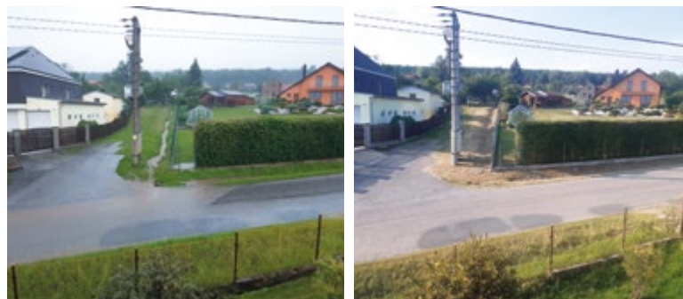
Fig. 3. Situation in the area of piping and canalization of a small stream below the main road in the village of Drahlín during the flash flood in June 2024 compared to standard situation at the end of August of the same year
