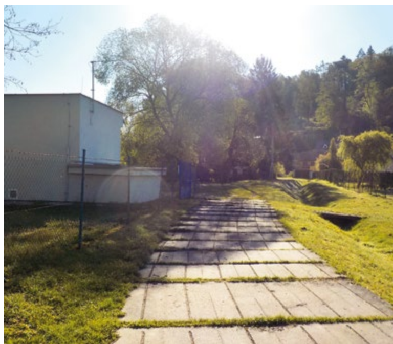
Fig. 6. Groundwater abstraction facility at Tupadly in the Liběchovka catchment
