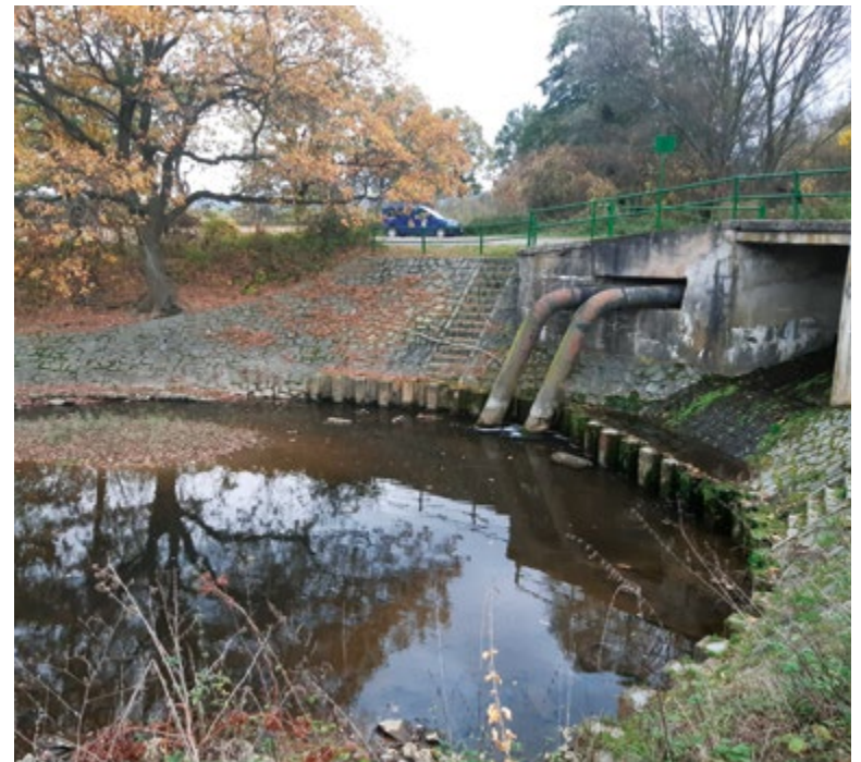
Fig. 8. Current situation below Bojmany weir at the spillway for the riverbed, which was used to supply the disappeared pond system and now returns behind the weir to the Doubrava river (November 2023)
