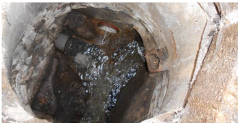
Fig. 2. Example of a sampling point on sewage connection (Source: TGM WRI archives)
