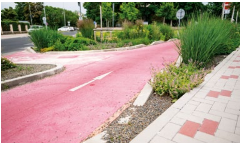
Fig. 1. Rain gardens line the pavements and roads in Roudnice nad Labem (Source: Nadace Partnerství – Adaptterra Awards, photo: V. Herout)
