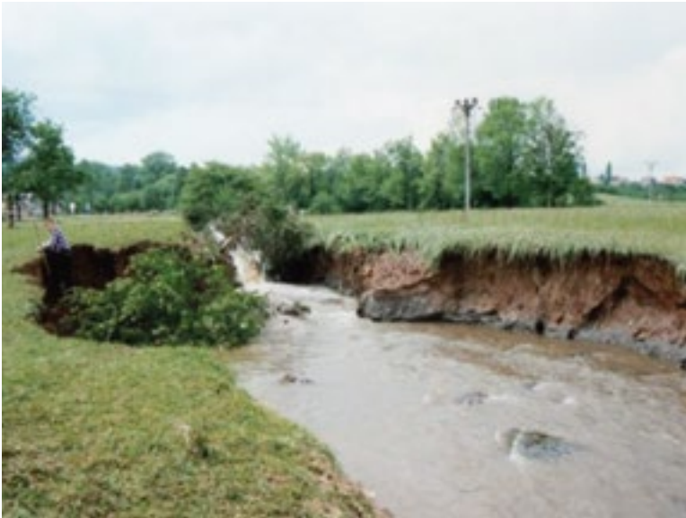
Fig. 1. Development of the „pear shaped“ scour resulting from degradation of a drop structure on flash flood (left); feature of flow in transitional zone of the spatial 3D scour (right)
