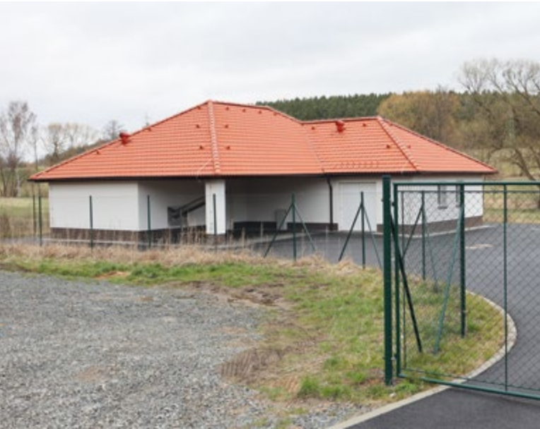
Fig. 2. Ledce municipality – WWTP 1,000 PE with sewerage (Photo: T. Homola)
