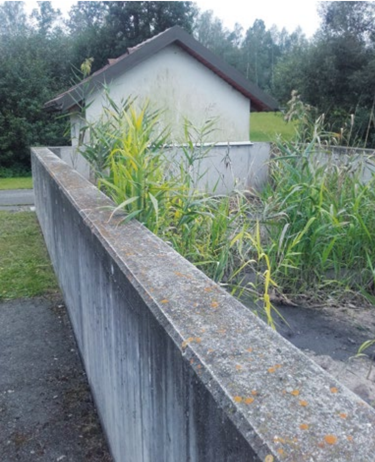
Fig. 2. STRB unit for village WWTP, size below 200 p.e., Austria
