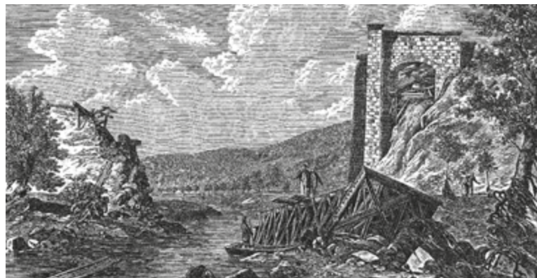
The destroyed bridge of the Buštěhrad Railway, the flood of 1872
