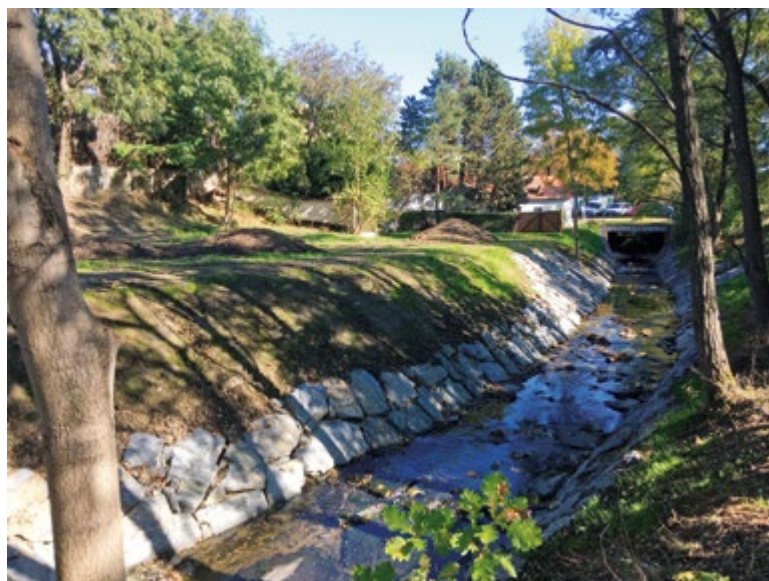
Fig. 6. Restored part of Kunratický stream below Vrbova street
