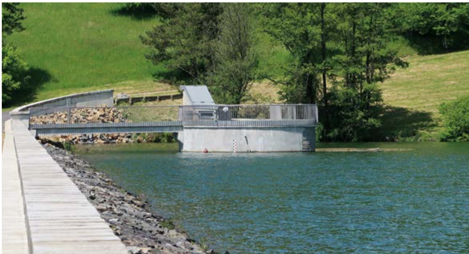
Fig. 3. Ludkovice water supply reservoir
