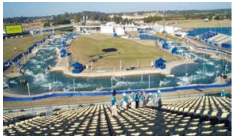
Olympic Games 2000 in Sydney, Jaroslav Pollert st. – design and implementation of an artificial runway for water slalom, stadium layout
