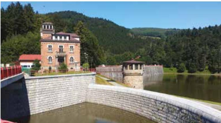
Fig. 5. Bystřička hydraulic structure completed in 1912, safety spillway
