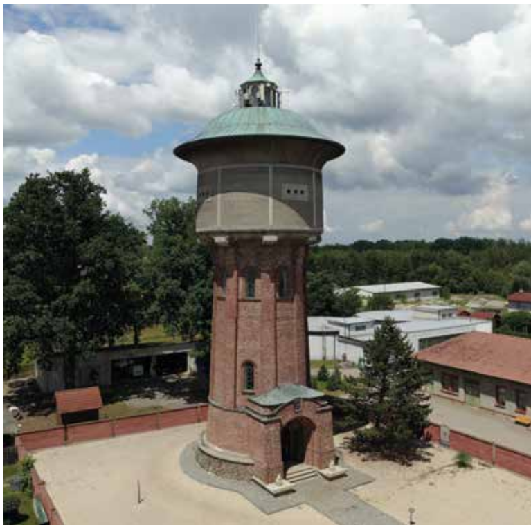
Fig. 6. The shape of the elevated water tank in Třeboň was designed by architect Jan Kotěra, who was also in charge of the design of the elevated water tank of Vršovice waterworks in Prague-Michle (Photo: O. Cívín)
