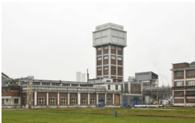
Fig. 15. The elevated water tank in Ostrava-Mariánské Hory is united with the surrounding buildings by a reinforced concrete skeleton with a combination of plastered surfaces, faced masonry, and openwork motifs (Photo: R. Polášek)
