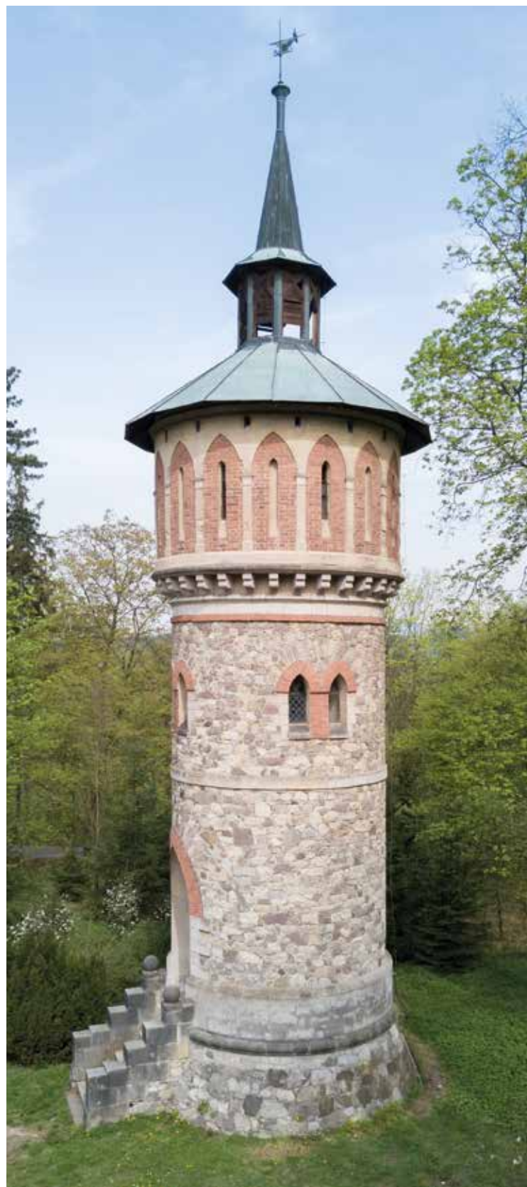
Fig. 20. An elevated water tank also formed part in the water supply of Sychrov Castle park, where the supporting structure on a circular ground plan was used in our territory for the first time (Photo: O. Cívín)
