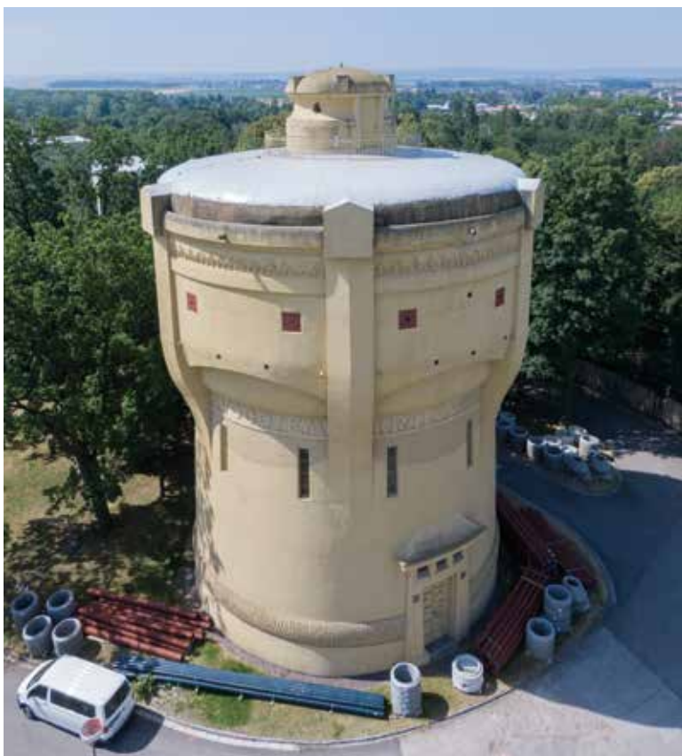
Fig. 7. The oldest preserved reinforced concrete elevated water tank in an urban environment was built in Pardubice in 1907 (Photo: O. Cívín)
