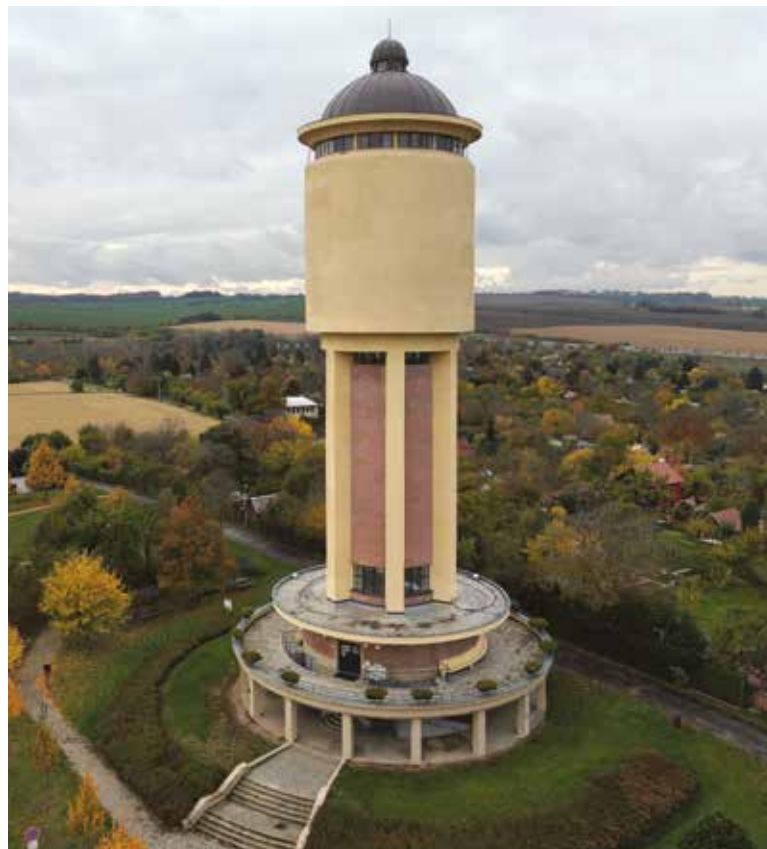
Fig. 8. Elevated water tank in Kolín, designed by architect František Janda in a functionalist style (Photo: O. Cívín)
