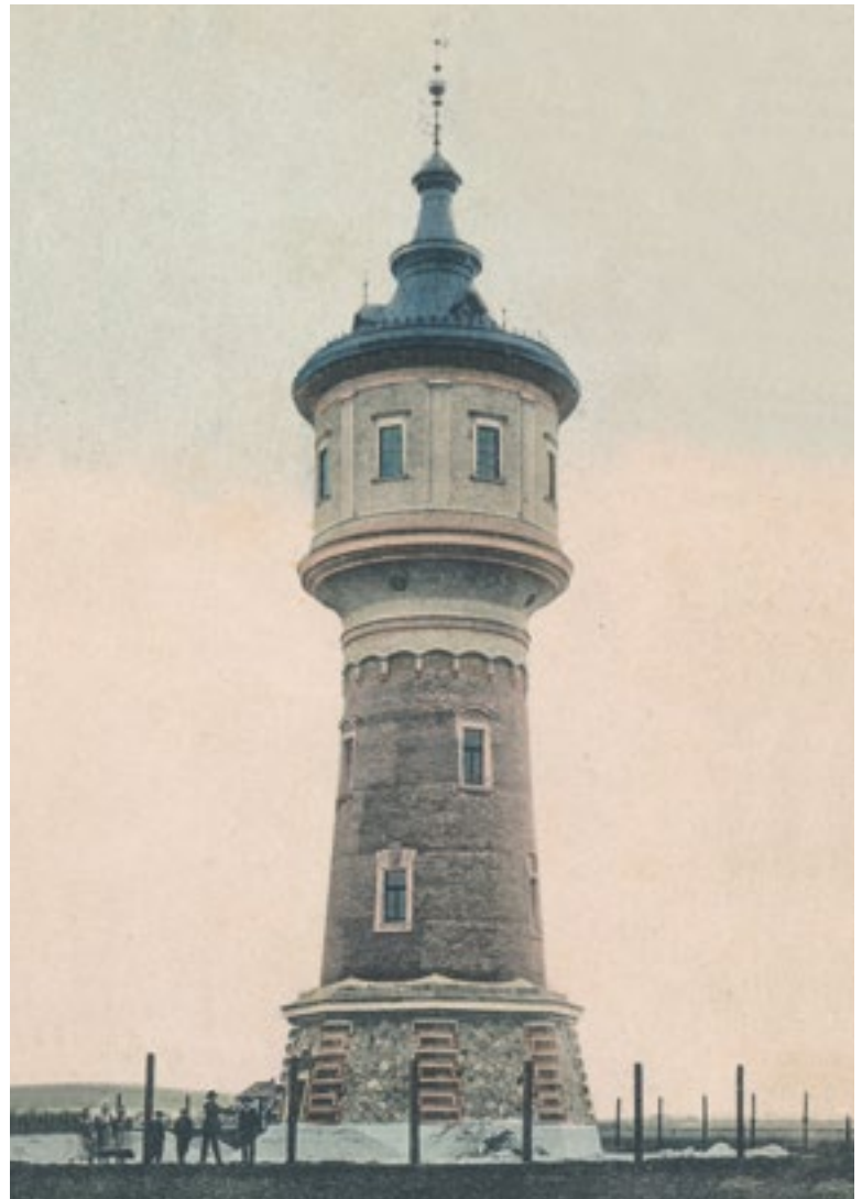
Fig. 5. Libeň elevated water tank from 1904, with the characteristic extension of the shell around the Intze reservoir (Archive of R. Kořínek)
