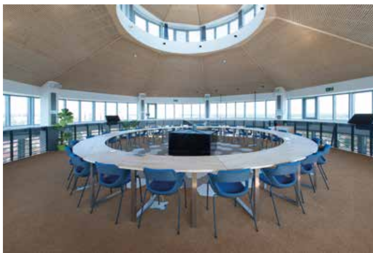
Fig. 24. The elevated water tank in Kladno from 1933 underwent a challenging conversion and its top floor today serves as a meeting room for the local waterworks company (Photo: M. Vonka)
