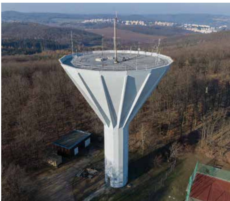
Fig. 22. The elevated water tank found in Brno-Kohoutovice since 1969 was designed by the architect Tomáš Čeroušek (Photo: O. Cívín)
