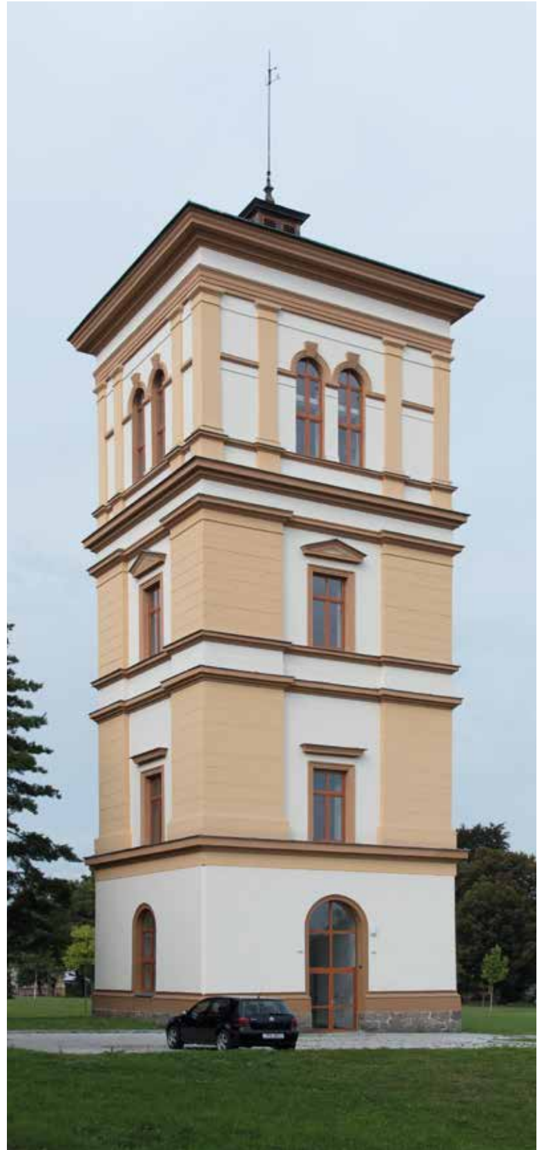
Fig. 18. The elevated water tank of Dobřany psychiatric hospital was built at the time of the construction of the hospital between 1876 and 1883 (Photo: R. Kořínek)
