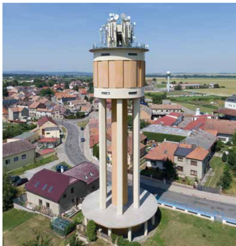
Fig. 9. Combined load-bearing structure of the elevated water tank in Chrast (Photo: O. Cívín)
