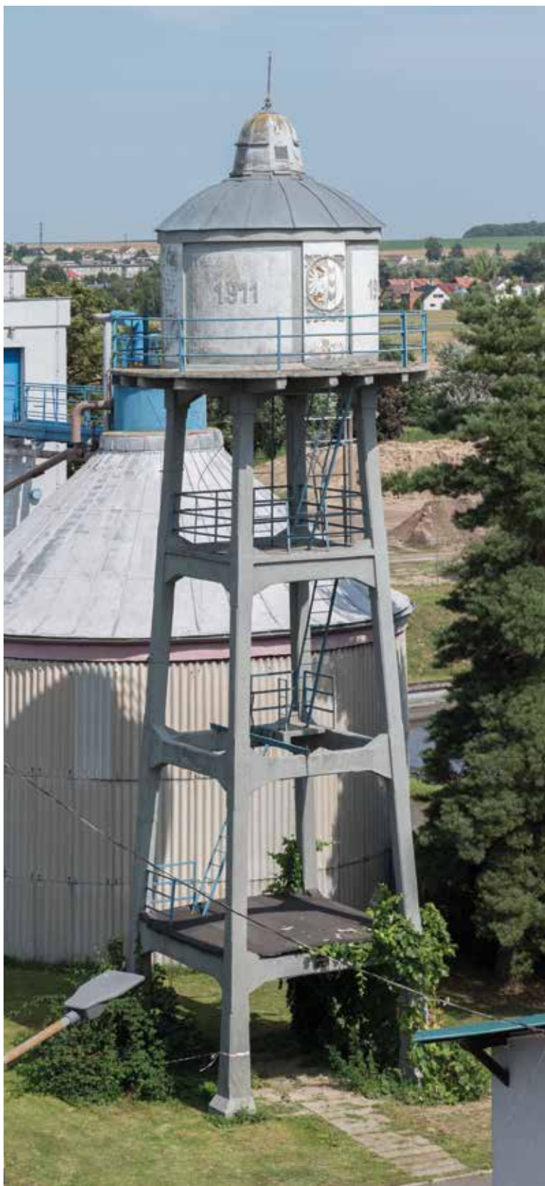
Fig. 19. Open reinforced concrete supporting structures were used in our territory for the first time for the construction of the elevated water tank of Opava wastewater treatment plant (Photo: R. Kořínek)
