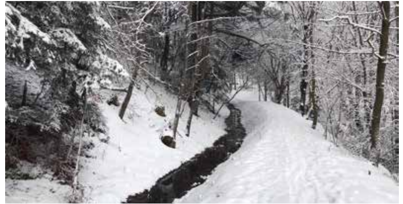
Fig. 7. Collecting ditch after restoration by CA (Photo: S. Červeň)
