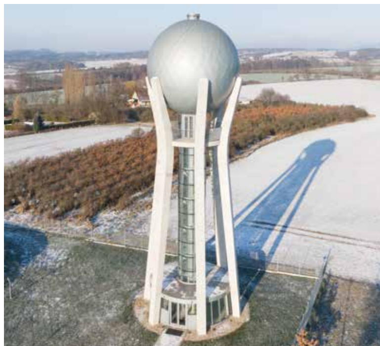
Fig. 23. The shape of the elevated water tank in Ohrazenice proves that it still makes sense to look for original and decent solutions for these structures (Photo: O. Cívín) [25]
