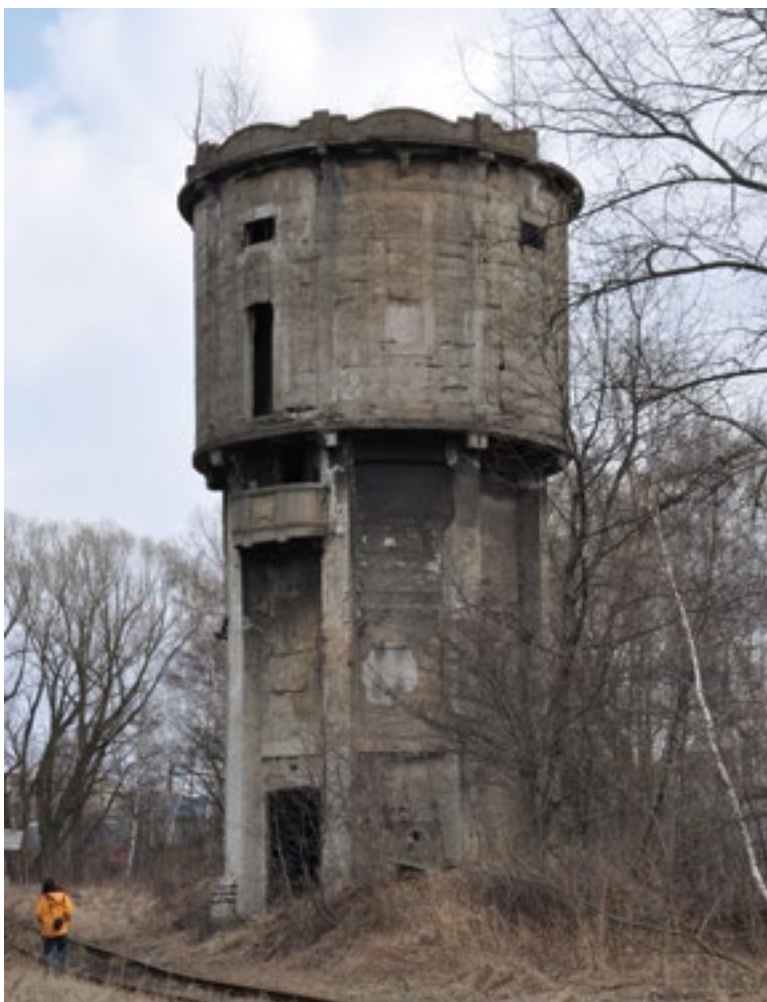
Fig. 3. Bohumín elevated water tank is the first documented example of the use of reinforced concrete for these railway structures (Photo: R. Kořínek)
