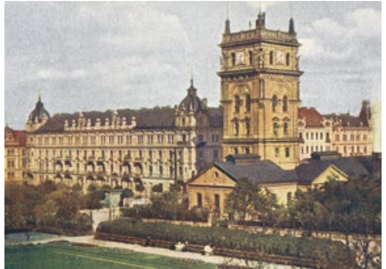
Fig. 4. The Neo-Renaissance elevated water tank of the former Královské Vinohrady aqueduct is still a prominent feature of this part of the city of Prague (Archive of R. Kořínek)
