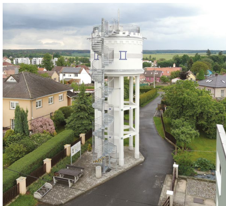
Fig. 13. The reinforced concrete elevated water tank in Heřmanova Huť – Dolní Sekyřany was rebuilt as a lookout tower and is accessible to the public (Photo: O. Cívín)
