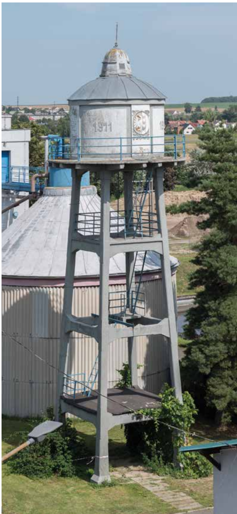
Fig. 19. Open reinforced concrete supporting structures were used in our territory for the first time for the construction of the elevated water tank of Opava wastewater treatment plant (Photo: R. Kořínek)
