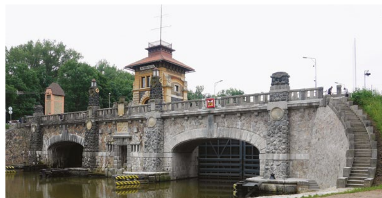
Fig. 7. Hořín lock, new moveable bridge (Photo: O. Hrdlička, 2021)
