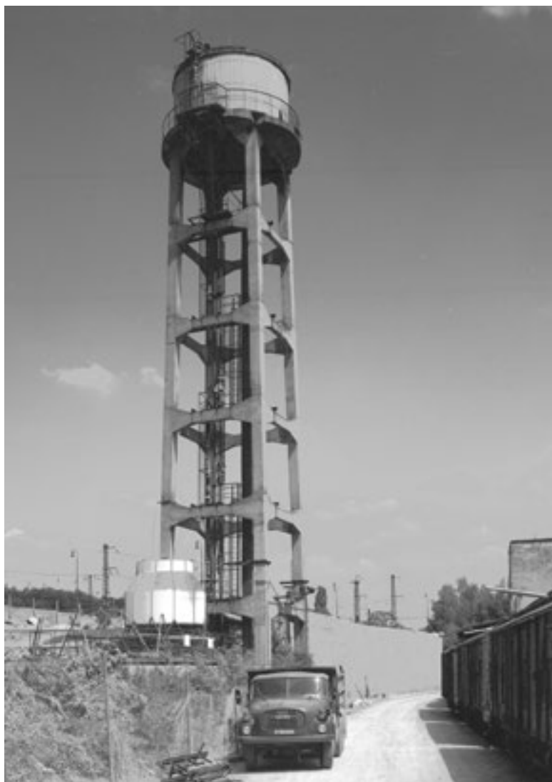
Fig. 14. An elevated water tank for the Michelin tyre factory in Prague-Záběhllice was built in a purely utilitarian style [21]
