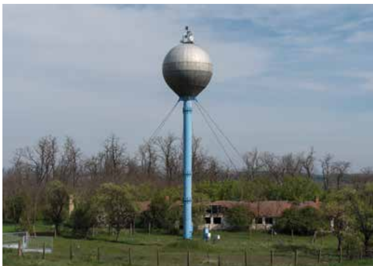
Fig. 21. The first Hydroglobe elevated water tank in our territory was built in Borotice (Photo: R. Kořínek)
