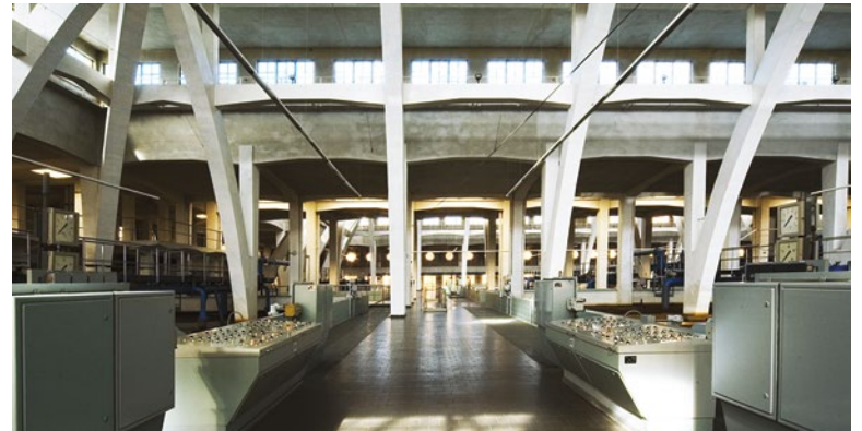
Fig. 3. Prague Podolí water treatment plant, filtration hall, current condition (Photo: PVK Archive, 2018)
