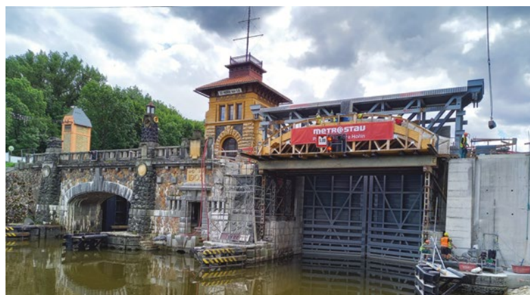
Fig. 6. Hořín lock, new moveable bridge (Photo: O. Hrdlička, 2021)
