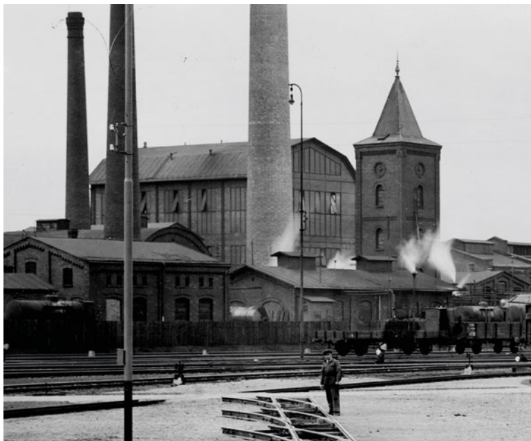
Fig. 10. One of the first elevated water tanks built in industrial complexes was Rudolf Rütgers's tar processing plant in Zábřeh nad Odrou (today part of Ostrava) [19]
