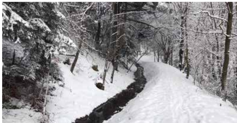
Fig. 7. Collecting ditch after restoration by CA (Photo: S. Červeň)
