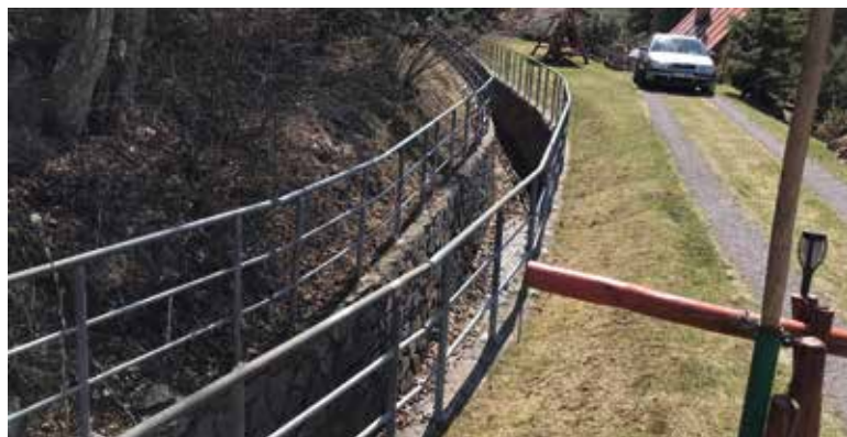
Fig. 9. Inappropriate reconstruction of one of the collecting ditches (Photo: S. Červeň)
