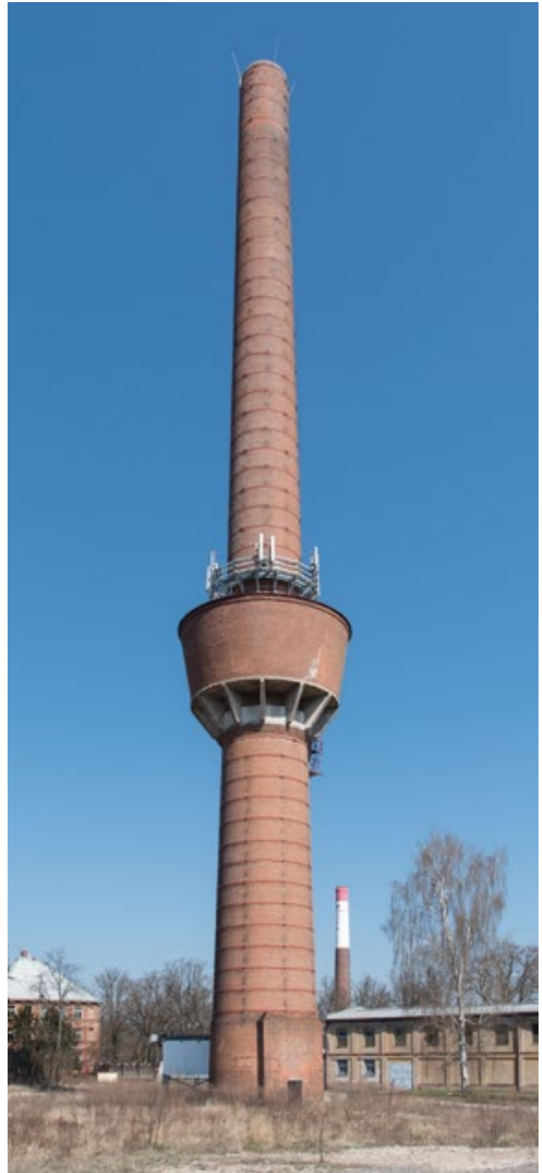
Fig. 16. In 1942, an 80-metre high chimney with a reinforced concrete reservoir with a volume of 300 m 3 was built for Josef Sochor's Mechanical weaving and textile printing works in Dvůr Králové nad Labem (Photo: M. Vonka)
