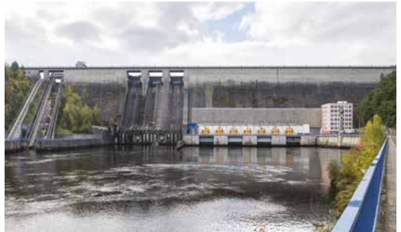
Fig. 6. Orlík hydraulic structure, concrete gravity dam completed in 1960 (Photo: V. Macha, 2021)
