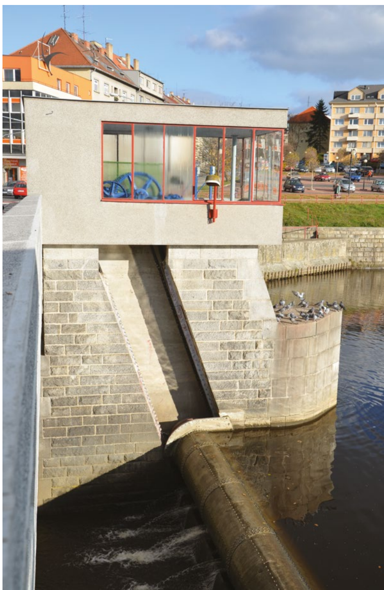
Fig. 10. Písek, New bridge, cylindrical weir, and hydroelectric power station, overall view (Photo: Z. Kohlíček, NPÚ, ÚOP České Budějovice)
