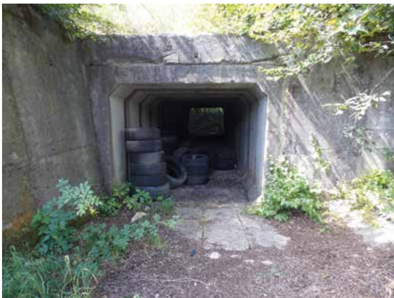
Fig. 8. Used tyres dumped in the outflow corridor downstream from DR safety spillway – Všemina II (AQUATIS, a. s.)
