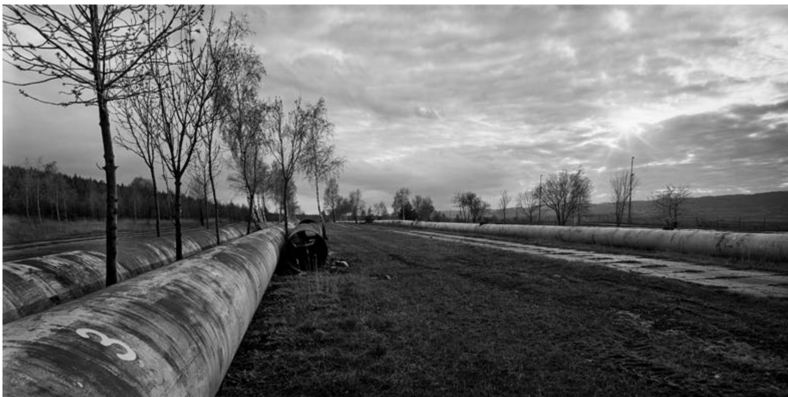
2018 – Along the Ervěnice Corridor, the Bílina river flows in pipes for three kilometres, within sight of the Czechoslovak Army lignite quarry
