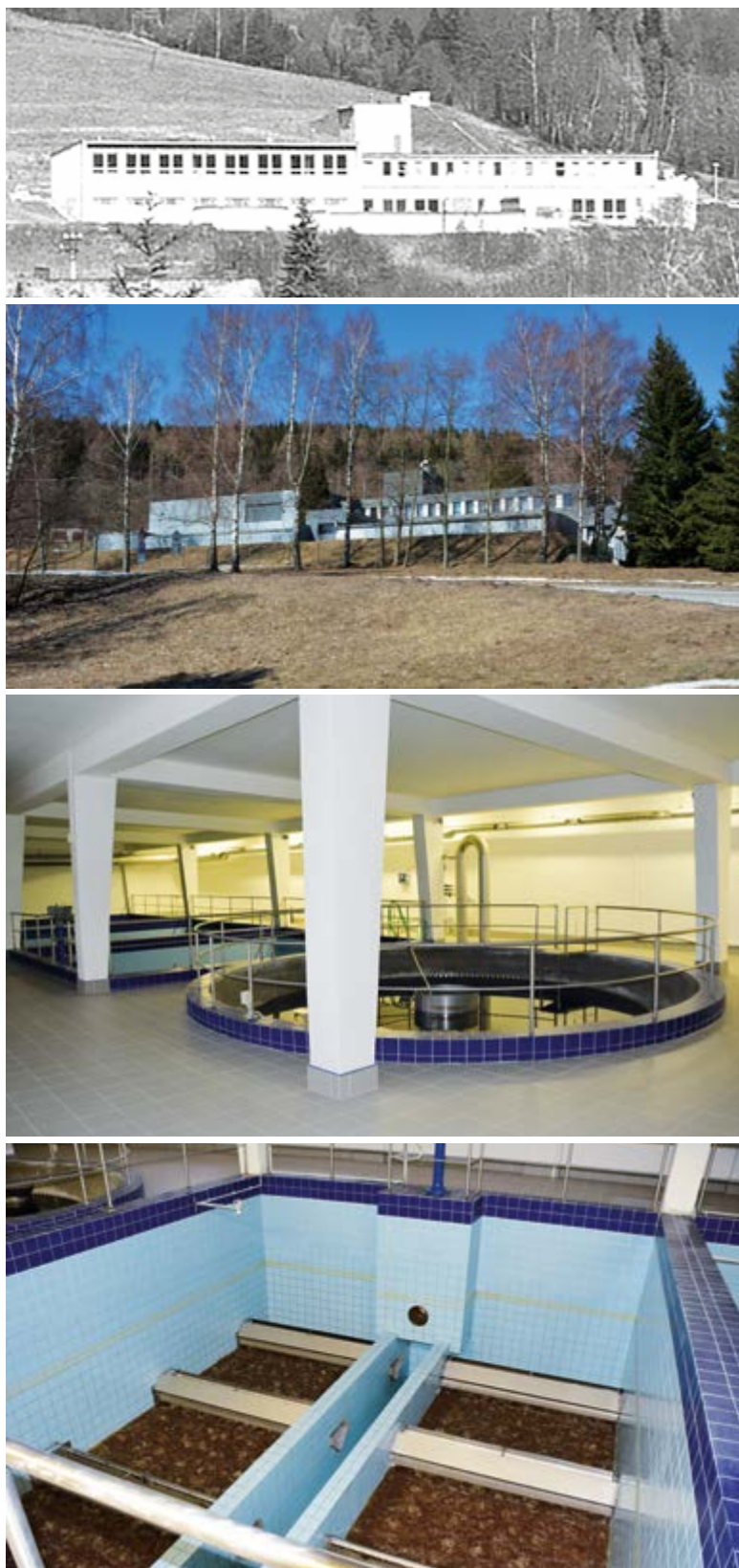
Fig. 5. Water treatment plant at the time of construction (ŠPVS archive), after reconstruction in 2008, the filters hall with reaction tank and filters, filter scrubbing (March 2022, A. Létal)
