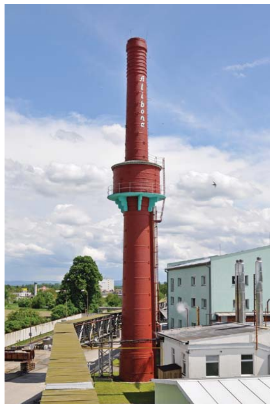
Obr. 6. Tovární komín s vodojemem v Litovli Fig. 6. Factory chimney with a water tank in Litovel
