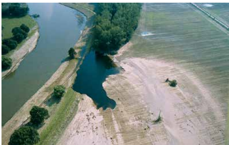
Fig. 1. Levee failure at the Mulde River (Saxony) during the flood 2002 (photo: Ott, 2002)
